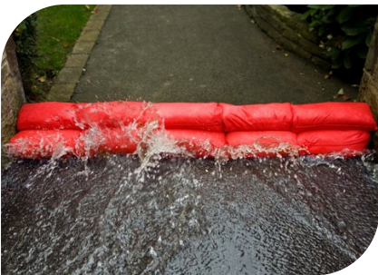
Gravitas International Ltd / Domestic flood control 2011 - water reactive sandbag / CC BY-SA 3.0
