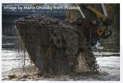
The material is typically removed by an excavator stationed in the stream or on the riverbank, and how it is disposed of will depend on the local area and the condition of the material.
