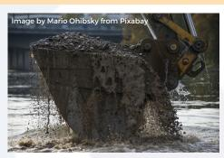
The material is typically removed by an excavator stationed in the stream or on the riverbank, and how it is disposed of will depend on the local area and the condition of the material.
