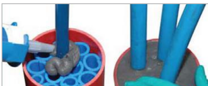
Sealant On Utility Entry Points
