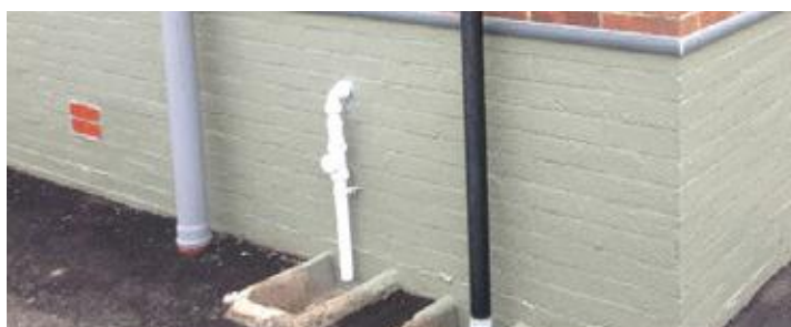
Non-Return Valve for Waste Pipes
