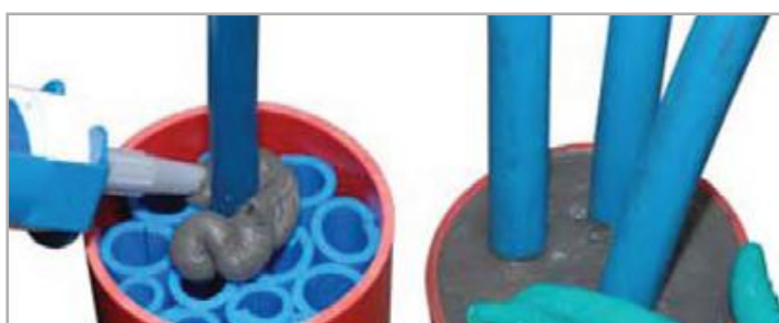
Sealant On Utility Entry Points
