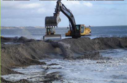
Beach refurbishment at Branksome Chine beach cc-by-sa/2.0 - © peter lloyd - geograph.org.uk/n/118179
