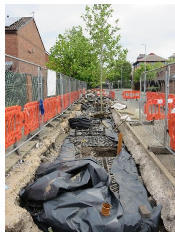
Installation of SuDS enabled tree trench, Salford
