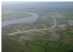
Image: The Environment Agency Hesketh Out Marsh West in the Ribble Estuary during the construction phase
