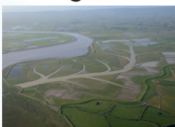
Image: The Environment Agency Hesketh Out Marsh West in the Ribble Estuary during the construction phase
