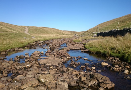
Cam Beck: over-widened, shallow channel
