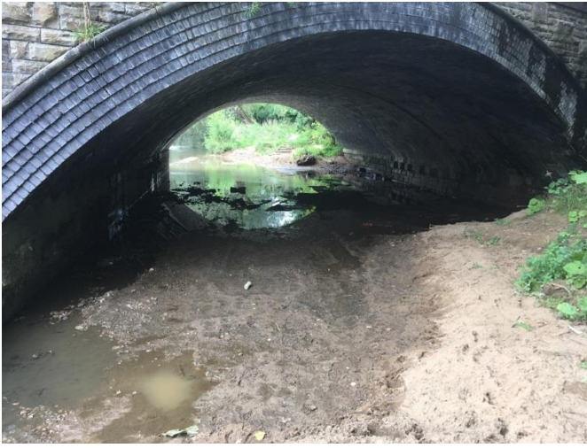
Padiham Bridge Gravel Removal - September 2018
