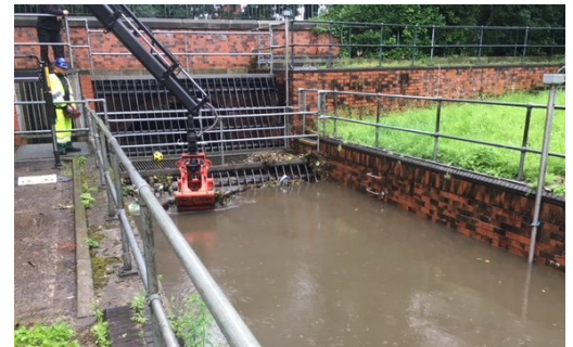
Clearing debris from river screen, south Manchester
