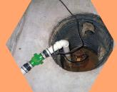
Sump pumps can be hardwired into mains electricity and also operate automatically.
