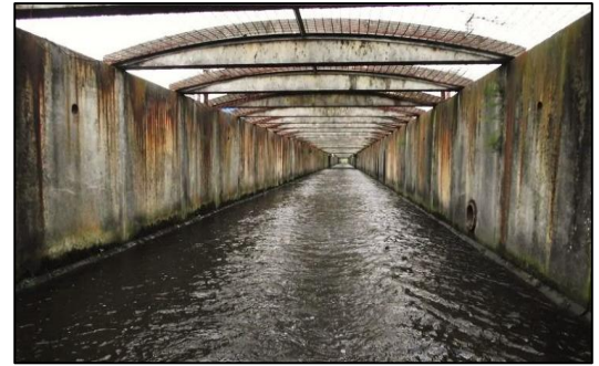
Figure 3: Knowsley Brook Culvert
