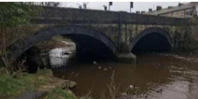
Gravel cleared from Padiham Bridge, March 2019
