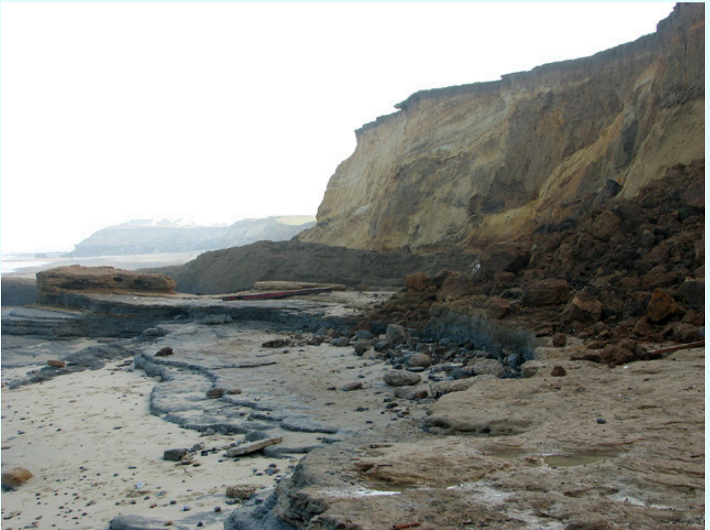
Storm Damage at Happisburgh - cc-by-sa/2.0 - © Evelyn Simak - geograph.org.uk/p/3774304
