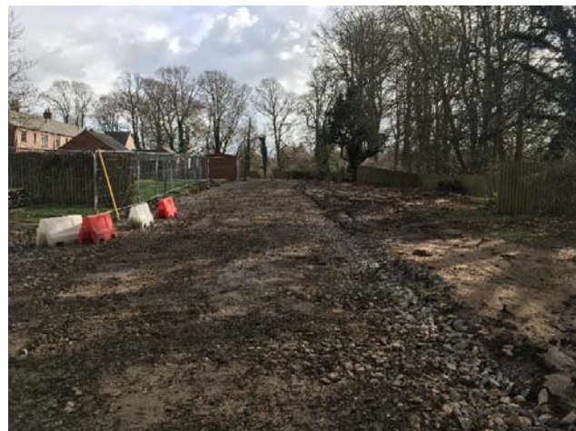
Above: Installed haul road at rear of properties
