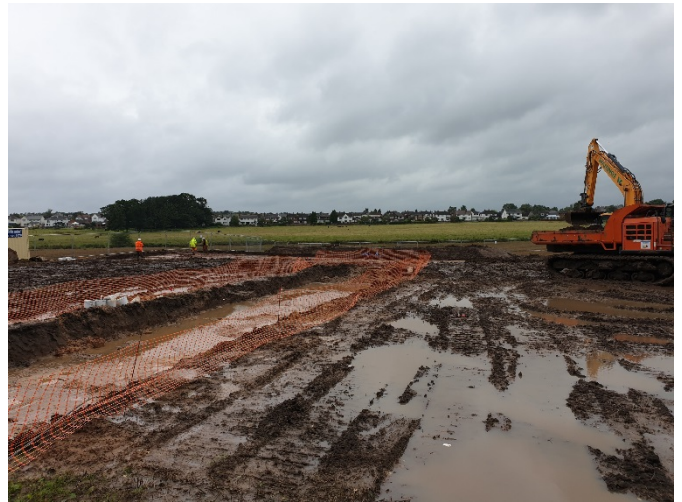
Above: Site compound set up
