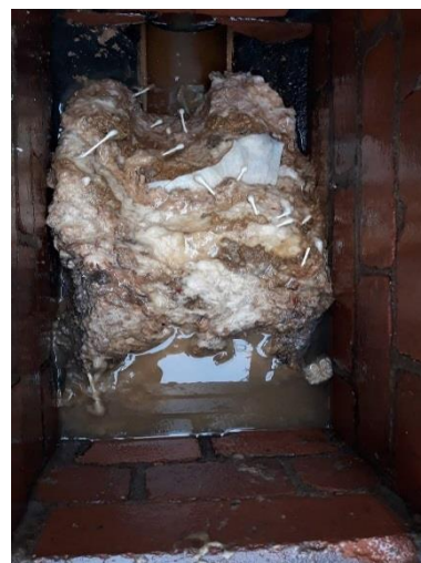
A recent blockage found in the UU sewer network – a mixture of cotton buds, wipes and kitchen roll. Only flush the 3p's!
