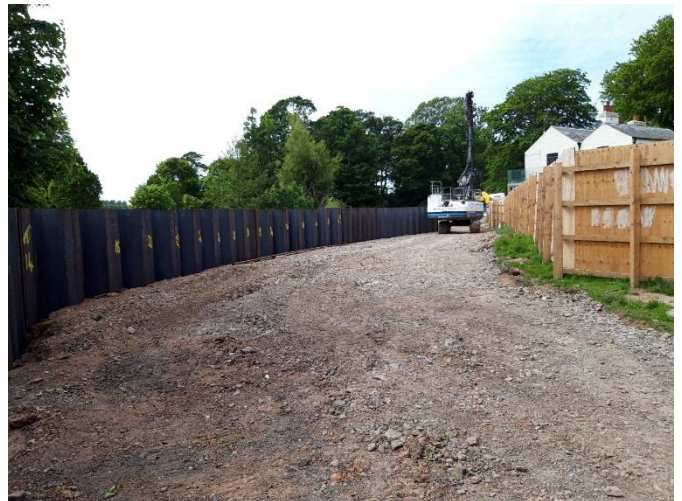
Above: Piling to the rear of Rickerby Retreat
