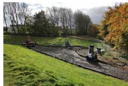
Works in Bitts Park underway
