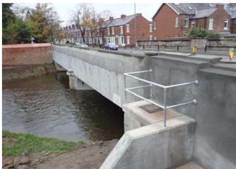
Botcherby Bridge improvements complete
