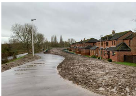
Riverside Way embankment and footpath
