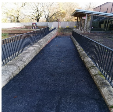
Sands Centre access ramp re-surfaced
