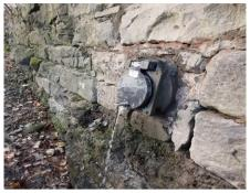
United Utilities have successfully installed flap valves to surface water outfalls off Riverside Drive which will help to manage the effect of backing up from high river levels.
