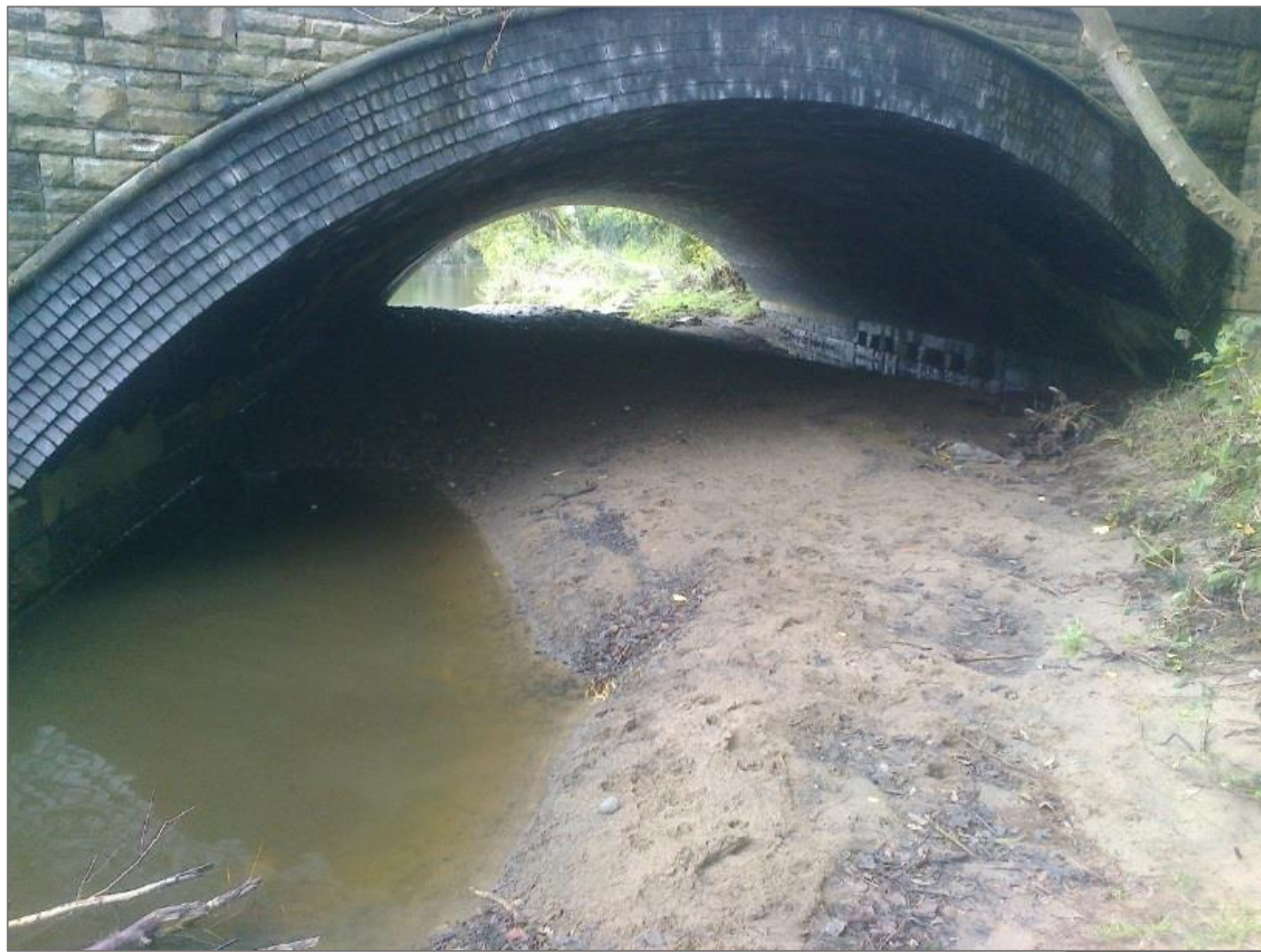
Gravel build-up under Padiham Bridge 23/10/17
