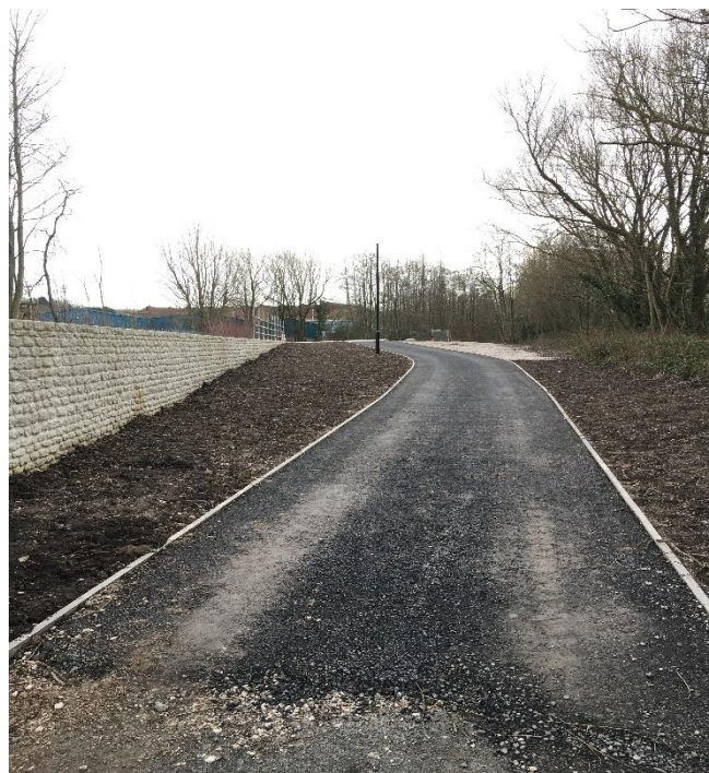
Re-surfacing of the new cycle path.
