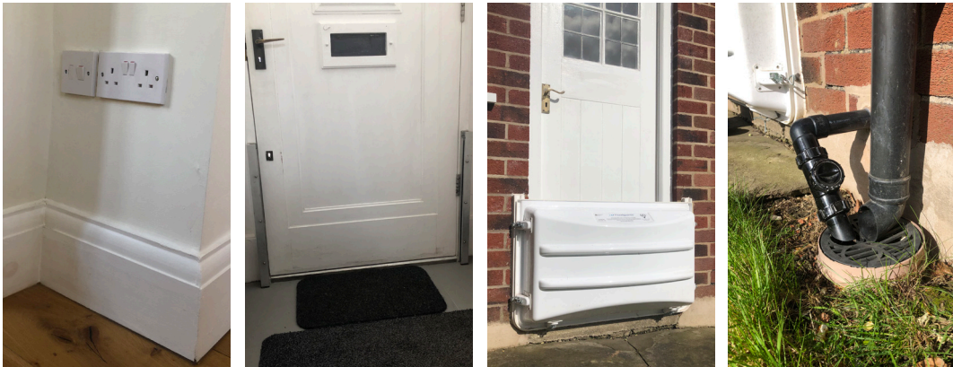
Electric sockets further up the walls, barriers to all external doors and non-return valves fitted.
