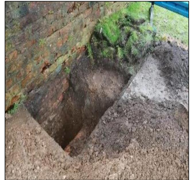
Hand dug trial pit
