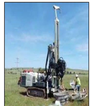
Sonic drilling rig
