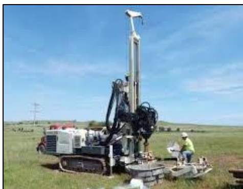
Sonic drilling rig
