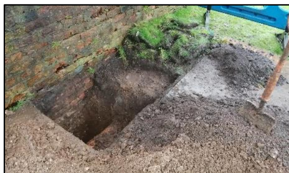
A hand dug trial pit
