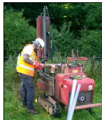
Window sample rig
