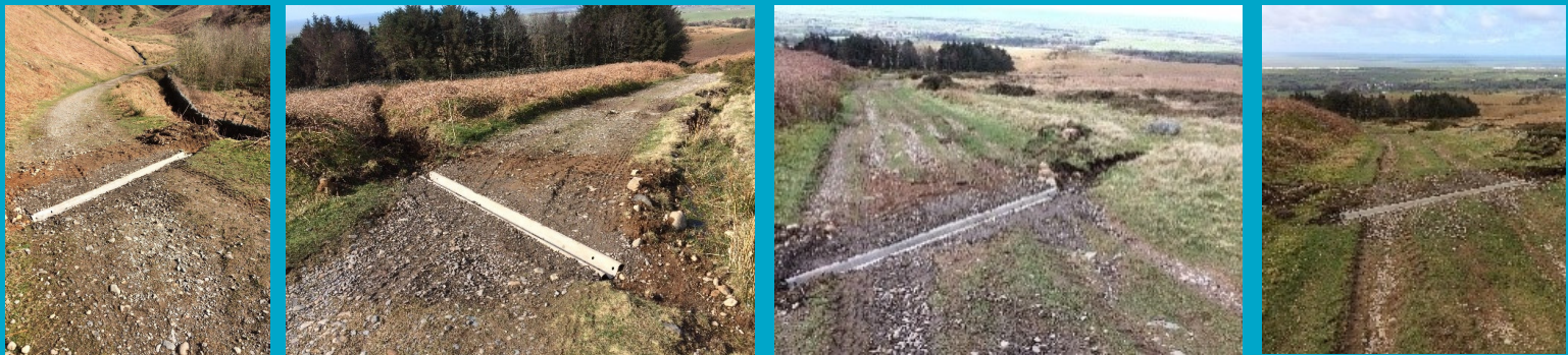
Images: West Cumbria Rivers Trust. Cross drains diverting runoff into surrounding vegetation
