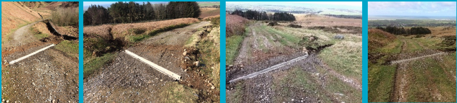
Cross drains diverting runoff into surrounding vegetation
