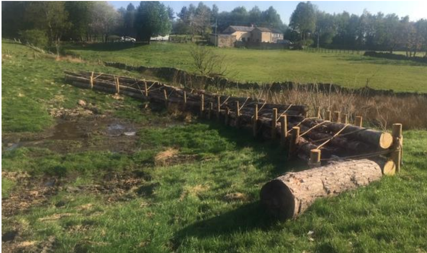
Engineered Log Jams. These pass forward low flows and attenuate high flows.
