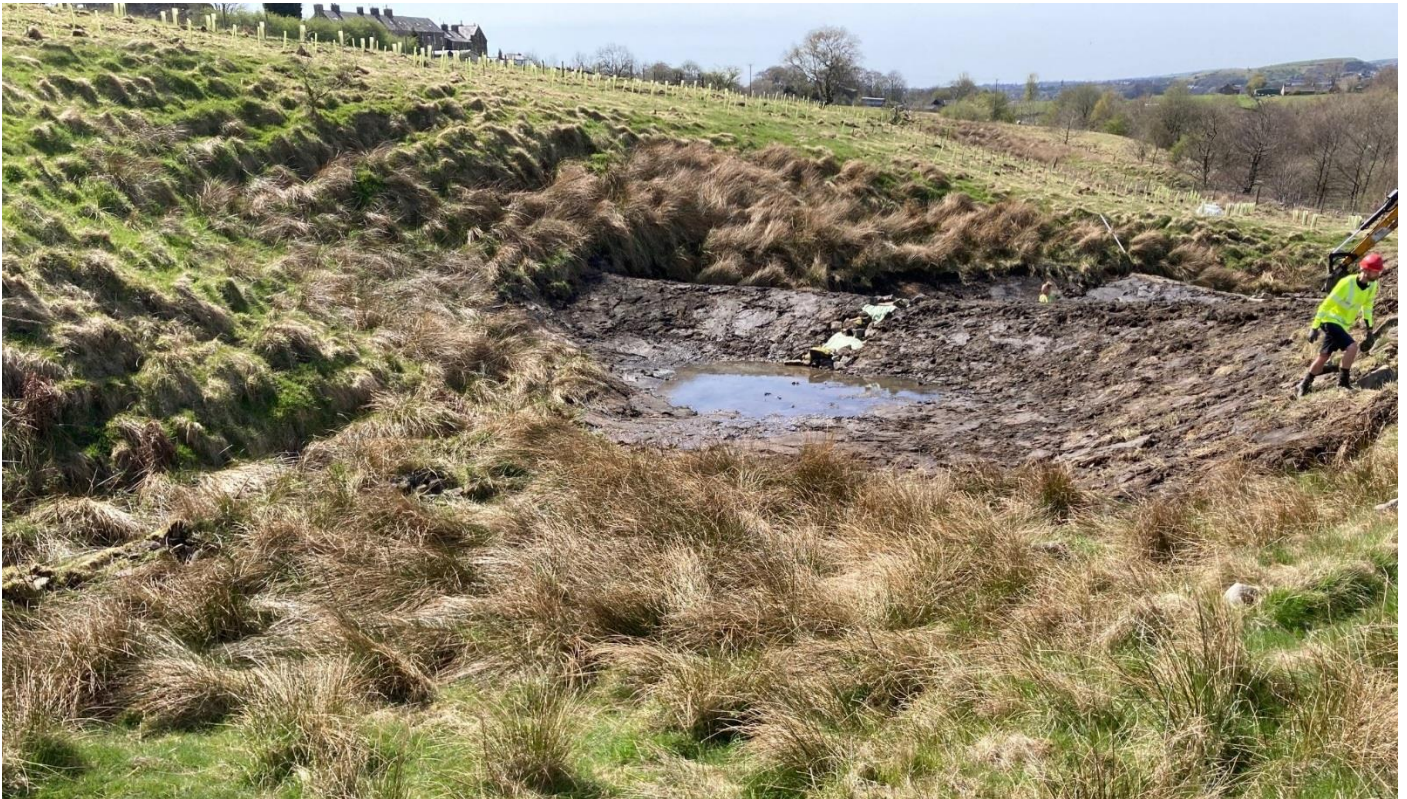
Large bunded barrier (with controlled outflow). These pass normal and low flows and fill and attenuate peak flows during storms.
