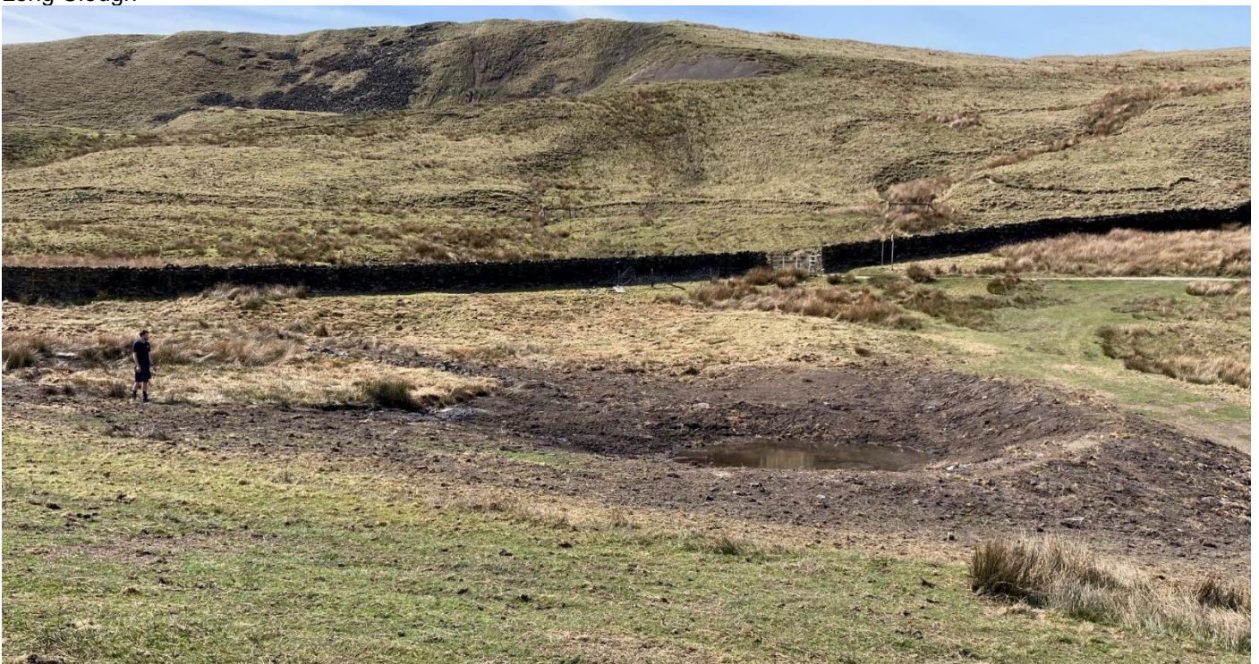
A series of 3 online bunded ponds up in the moorland headwaters with outflows, that pass low flows but attenuate storm flows.
