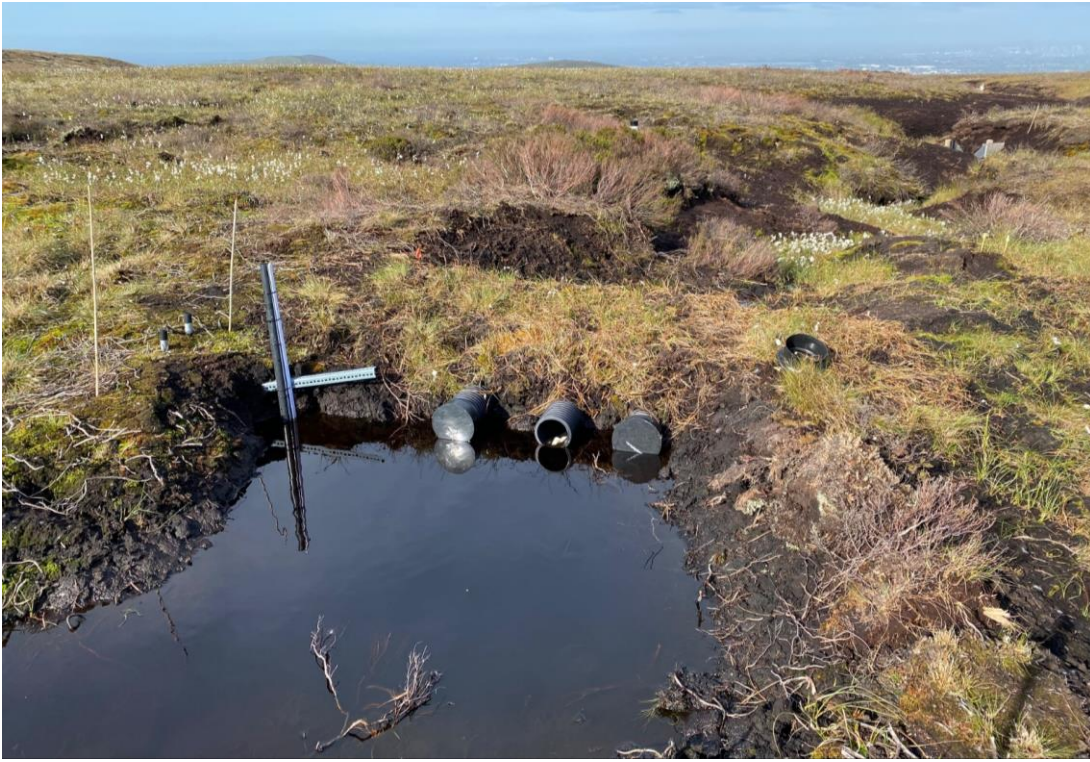
Piped peat dams
