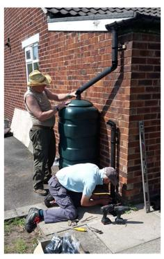
2. Water butts showing isolation valves and overflow pipe to raingarden
