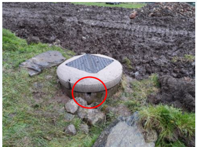
Photo of culvert before and after restriction placed on it (the outlet, as circled in red on the second image, can be amended following monitoring).
