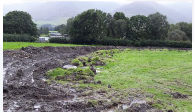
Photo of bund during construction.
