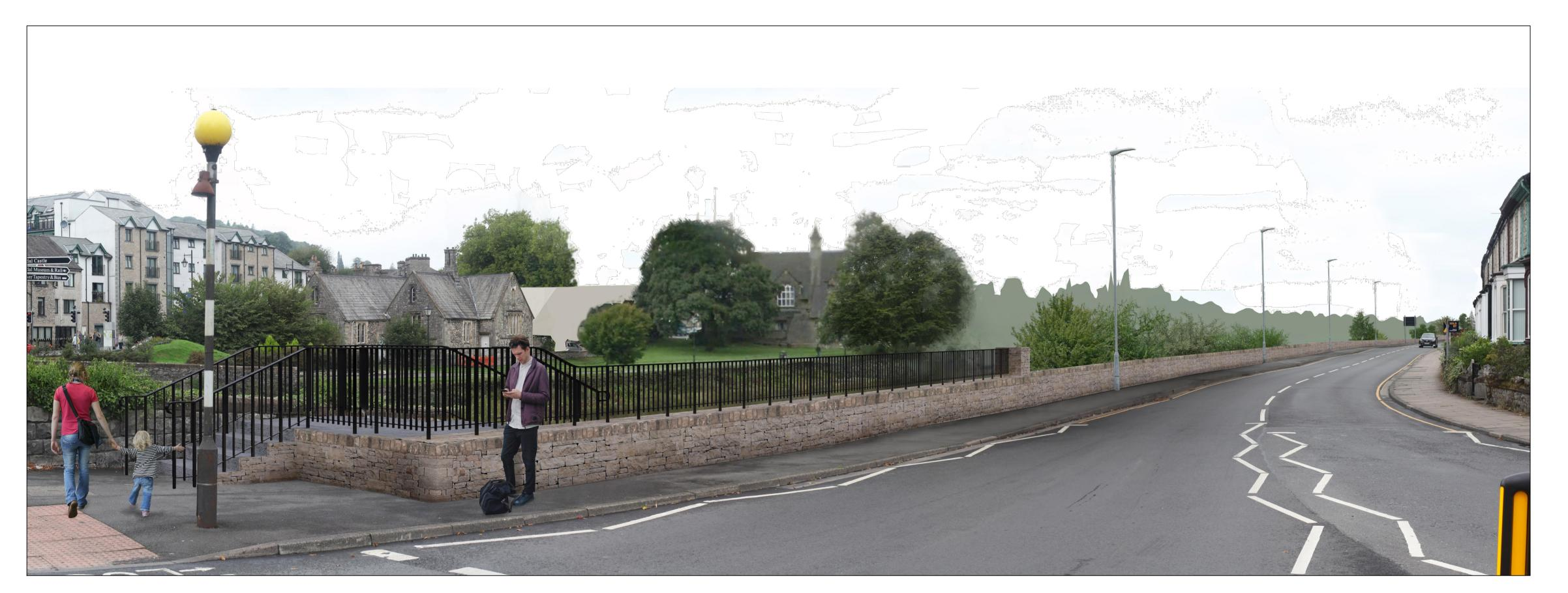
Proposed view illustrating all existing riverside trees cleared to facilitate works with flood defence wall. Up and over steps and railing to left of view and 600mm high wall mounted railing terminating in stone clad pier. Tree planting on regraded river bank visible above line of flood defence wall. Tree planting illustrated after 5year growth.
