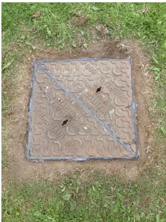
Fig 1: Manholes resealed at Green Lane & recreation field
