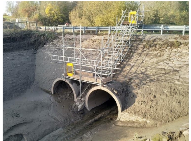
Existing Whittle Brook culvert investigation works
