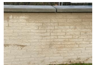
Imprinted brick used in one location to blend in with the local aesthetics
