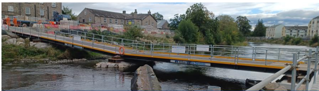
Temporary in-river bridge crossing and working platform
