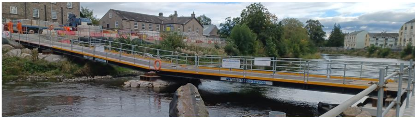
Temporary in-river bridge crossing and working platform
