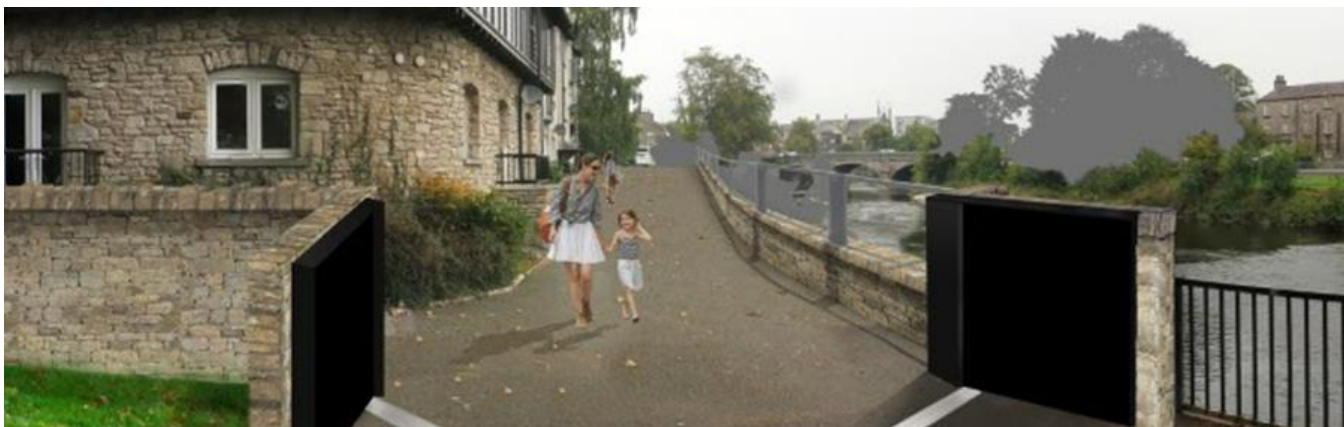
Proposed finish of the glass topped flood wall along Waterside
