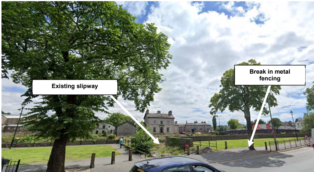
Figure 7 - New Road Common existing slipway and fencing arrangement
