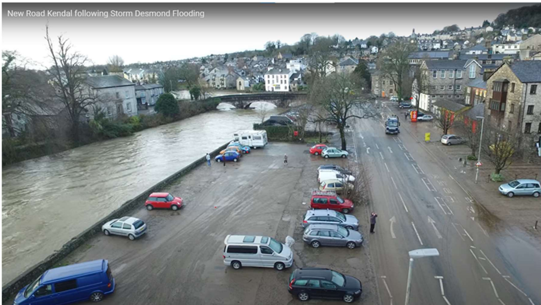
Figure 2 - Aerial photograph along New Road (facing west) on 6 December 2015 (Source - YouTube)
