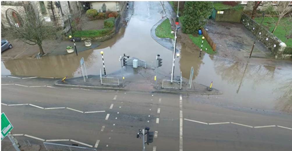
Figure 3 - Aerial photograph illustrating water ponding at junction of New Road (foreground) and Blackhall Road (background) preventing the throughflow of traffic along the one-way system
