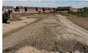
WALLASEY EMBANKMENT TOE REINFORCEMENT WORKS
