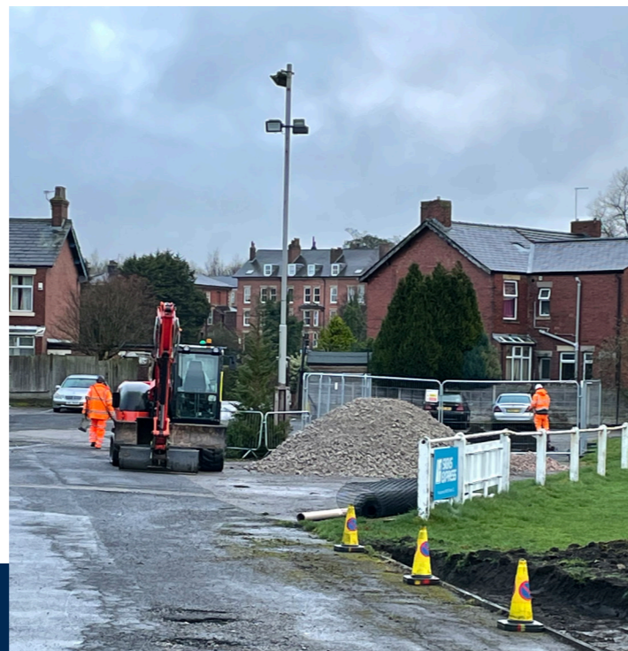
Through route construction at BAC/EE
