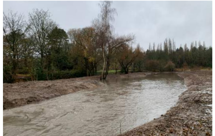
Completed pond during heavy rainfall
