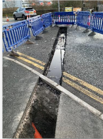
Site Investigation works undertaken in 2023 at Hardy's Gate Bridge
