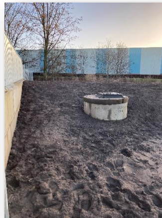
Finalised embankment tying in at Bury Point awaiting seeding
