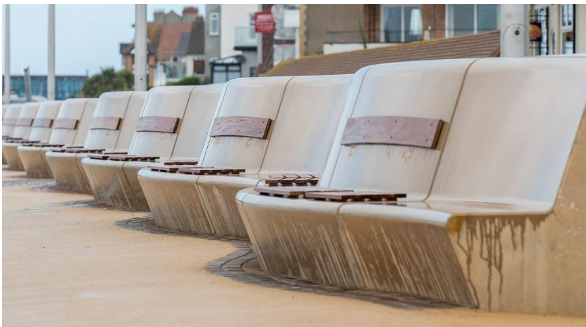
A section of the new flood wall at West Kirby
