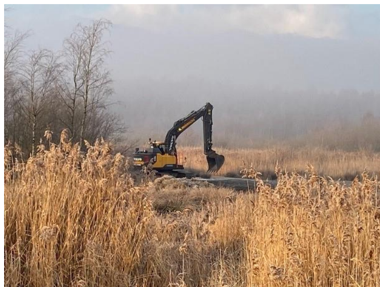
Figure 2: Digger in-situ creating wetland features.
