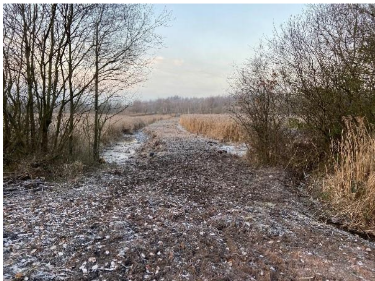
Figure 1: raised footpaths with newly installed culverts for water passage.
