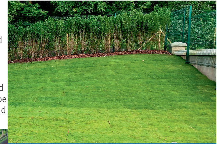
Completed fencing and hedge at the rear of Penwortham Methodist Church and the allotments
