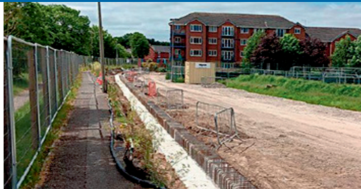
Foundations completed at the rear of BAC/EE
