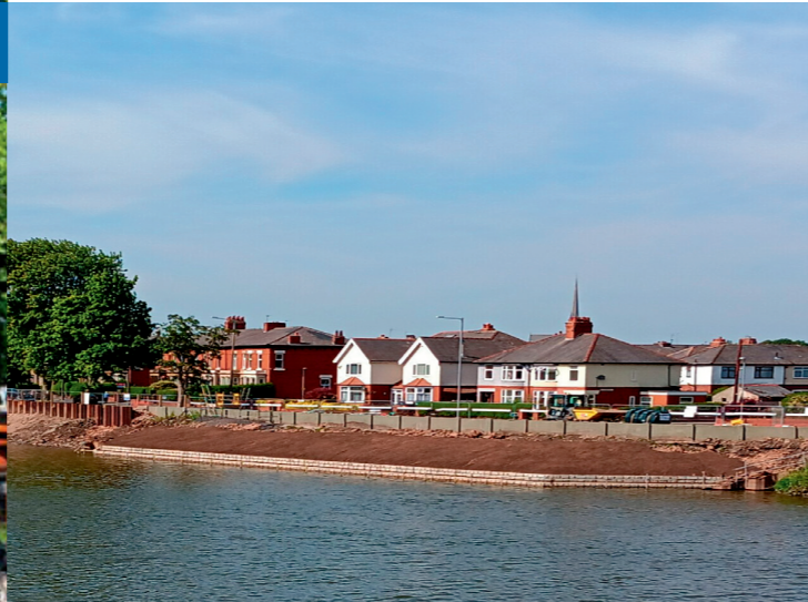
Piling taking place along Broadgate (left) and the Redi-rock revetment construction along the riverbank near Penwortham Old Bridge (right)
