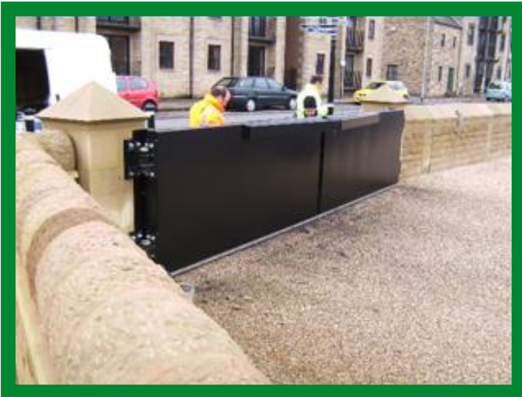
Example flood gate
