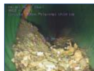
CCTV footage, damaged and blocked culverts
