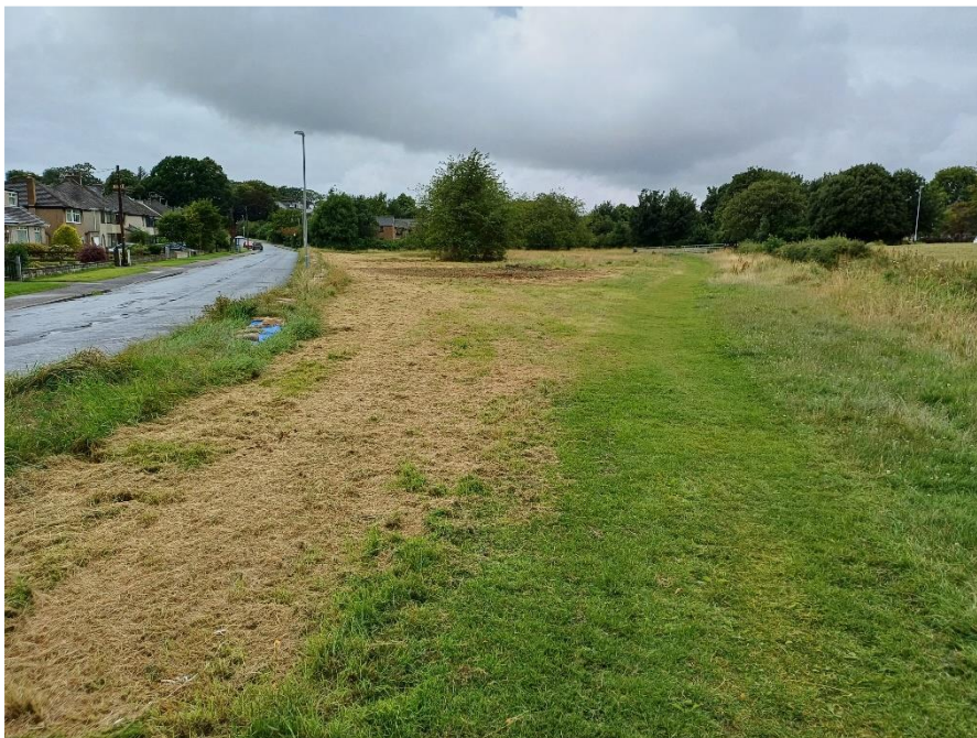
Image: View of cleared work area, looking from South to North
