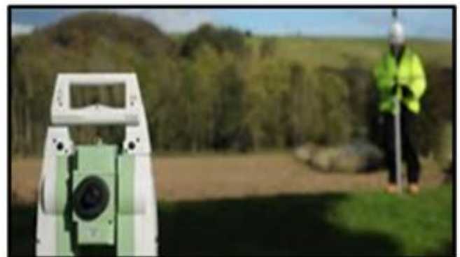
GPS laser and level equipment
